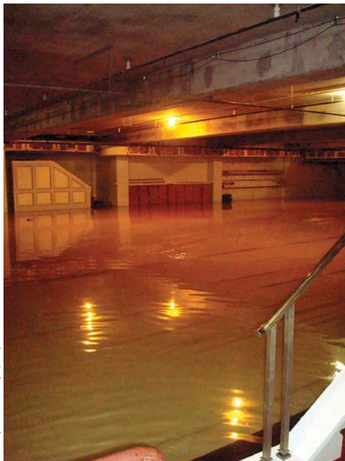
Flooding of the basement of the Nashville Symphony's Schermerhorn Symphony Center in 2010.
